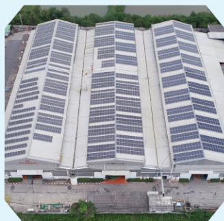
500 kW Ekarat Engineering Public Co., Ltd.
