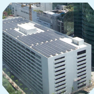
330 kW Energy Complex
